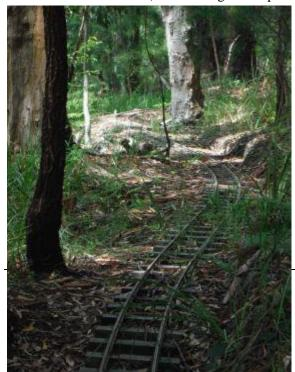
the USA similar miniature rail is most commonly supplied in 10 feet lengths. In general the longer the length the larger the gap between rail ends that must be left for thermal expansion and the more difficult is transport and handling. On the other hand shorter lengths mean more connections. Subject to minimum order quantities the rail can be made in any length up to 9 metres.
